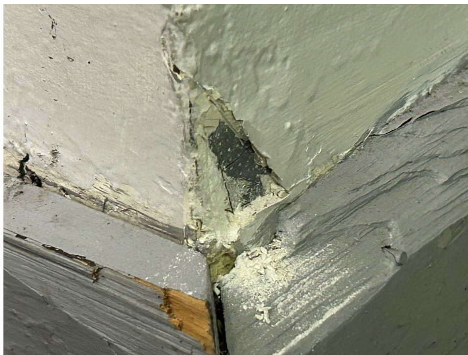
Photo 4 Non-asbestos drywall joint compound.
