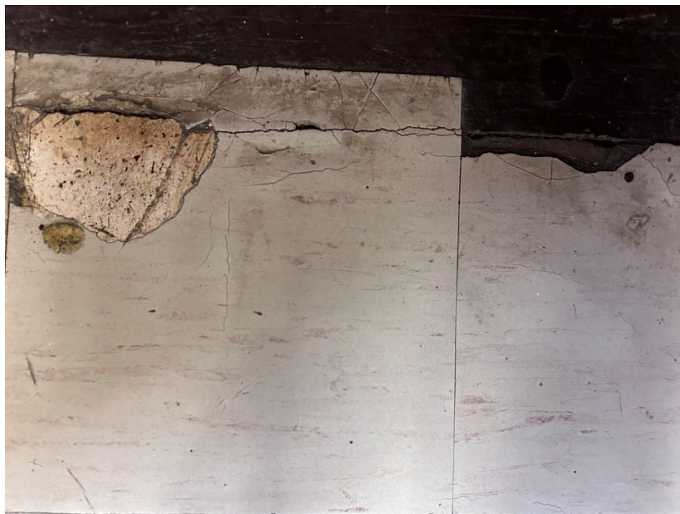
Photo 5 Non-asbestos 12" x 12" off-white vinyl floor tiles with faint burgundy streaks.
