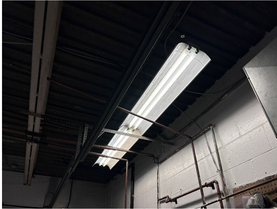
Photo 7 Mercury containing fluorescent light ballasts.
