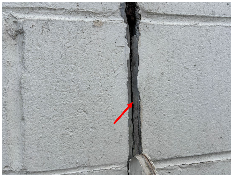
Photo 6 Asbestos-containing grey caulking.
