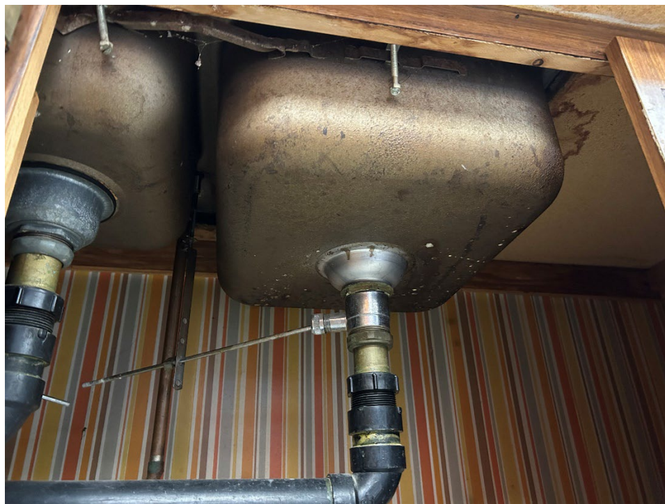
Photo 3 Asbestos-containing brown sink coating
